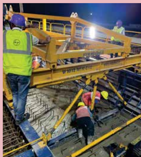
Rail construction in Bengaluru
