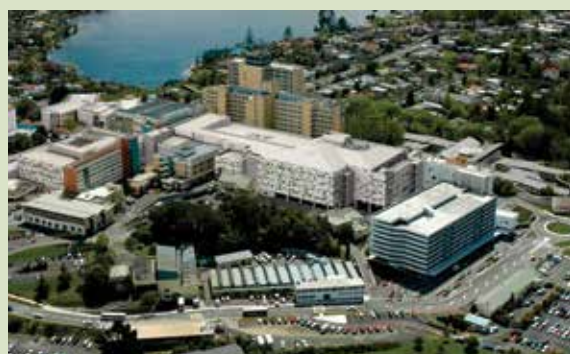
Aerial photo of Waikato Hospital
