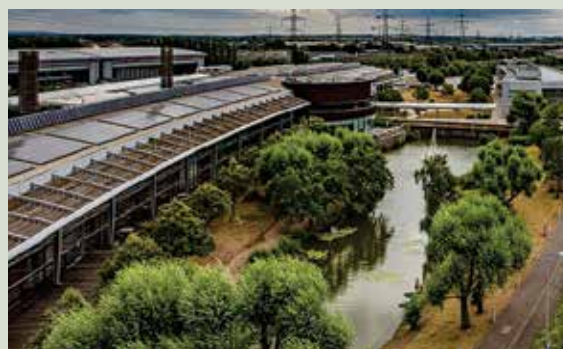
GEME campus created as part of redevelopment
